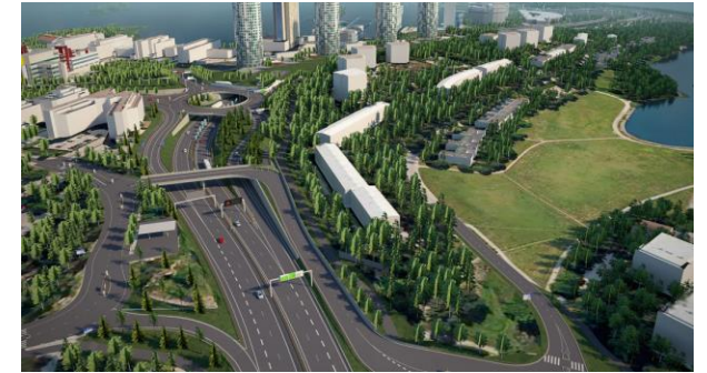
TUNNELS AND ROADS : Keilaniemi district and start of Ring I beltway
