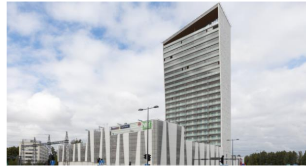
NEW CONSTRUCTION: Espoon Niittytorni complex high rise residential building
